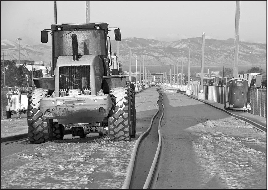
Denver RTD's East Rail Line after snowfall on February 26, 2014 between Peoria and Havana Streets near Union Pacific's Roydale (at right), looking west toward Denver. Welded rail had been laid for the two track line. – Photo © 2014 by Chip.
